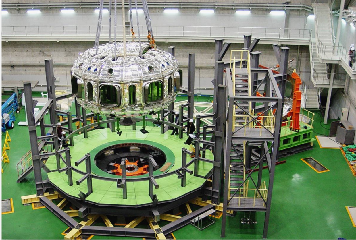
KSTAR VV and VVTS are installed in TKM Pit
